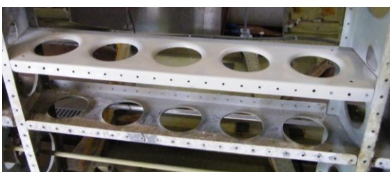
View of "cleaned up" frame section
